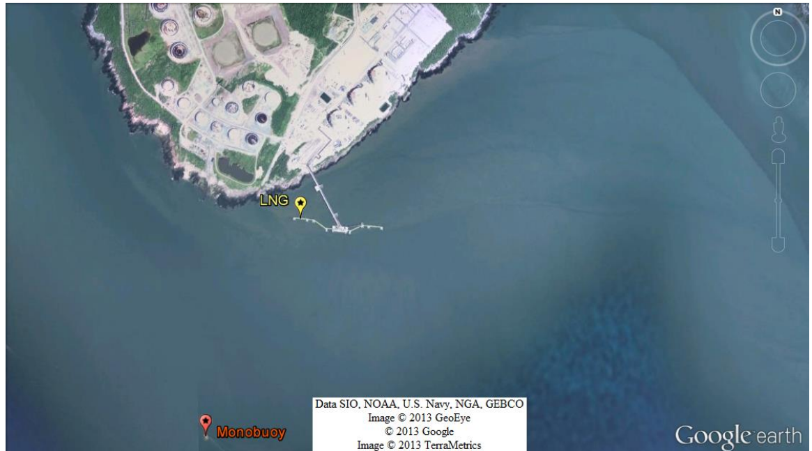
Figure 4. Location of recording equipment at the Liquefied Natural Gas (LNG) terminal study site. Crude oil tankers offload at the Monobuoy approximately 1 km away.
